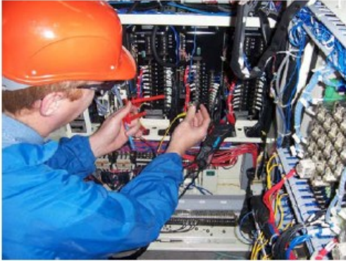
Fig. 9: Connecting in the MCC.
